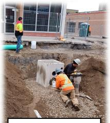
Setting and compacting around a new roadway catch basin
