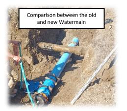
After another good week of construction, we are moving closer to being done the underground servicing work in the first stage of the Talbot Street Project. Remaining underground work includes Street lighting conduit, irrigation lines, storm catch basins, and the remaining Watermain and Sanitary building services.
